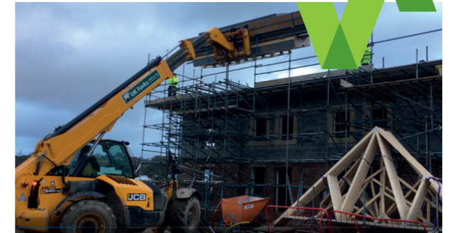
The site telehandler lifts the 3-4 packs onto the scaffold.
