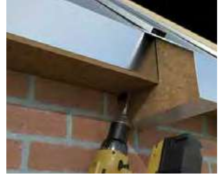
3. Add a fixing each side into the underside of the beam - use 4.2 x 38mm screw GPHS001
