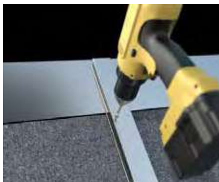
19. Fasten the clips, two into the roof panel and six into the ridge body using 4.8mm x 38mm screws GPHS001
