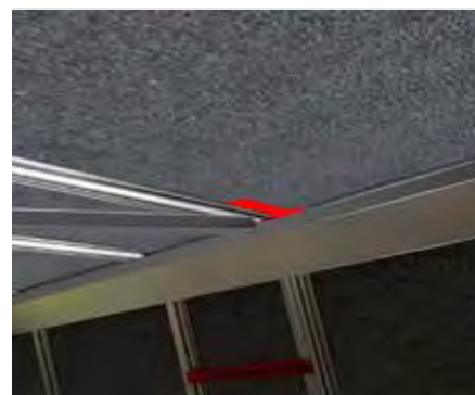
24. At the ridge 'spear' the long steel clip onto the roof panel rails, then drive/ tap the clip fully into the shelf before knocking the long clip fully onto the rails along its entire length. Then at the ridge end use four 5.5 mm x 19 mm screws HSBR001 to fasten through the shelf and into the steel clip
