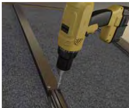
23. Now fasten the end of the short clip where it will abut the longer clip. Use two 4.2mm x 38mm screws GPHS001
