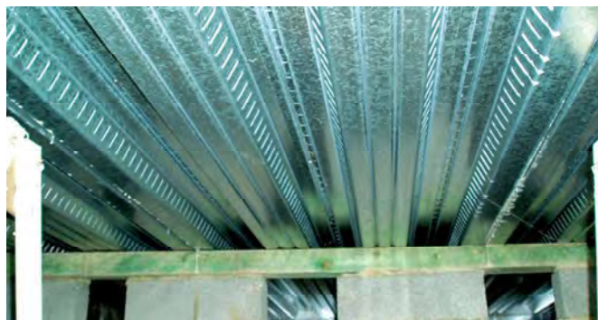
Figure 2 Galvanised steel decking supporting a suspended ground floor after 10 years exposure
