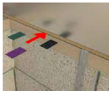
9. Where appropriate use packers supplied (varying thickness)
