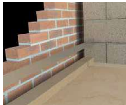
6. Offer up the 50 x 50 x 0.9mm steel angle onto the wall plate
