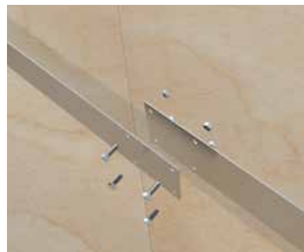
3. Take the two lengths of 2mm thick x 150mm steel tie plate and join together using the 4 x M10 x 25mm stainless steel nuts and bolts
