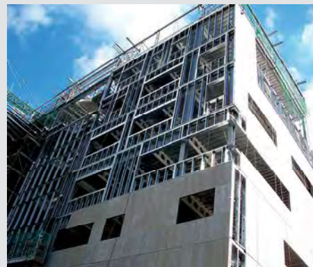
Light steel sections in an external wall application
