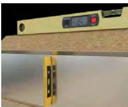
8. Now check beams are level and plumb – check dimensions against set out drawings
