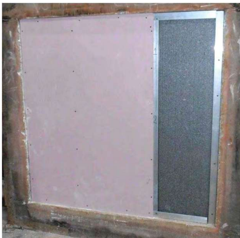
Photograph 6: Exposed face of Ultrapanel wall– during installation of 1 st (inner) layer of plasterboard.
