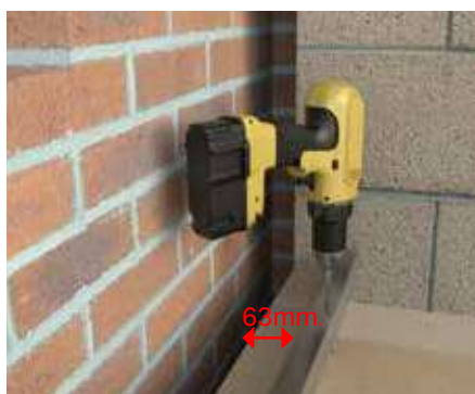
7. Measuring from the cavity side of the wall plate set the back edge of the angle plate inboard by 63mm. Screw down at 300mm centres using 4.2mm x 38mm screws (or 3.1 x 45 ARS nail)
