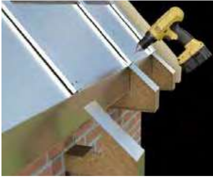
1. Add the soffit assemblies
