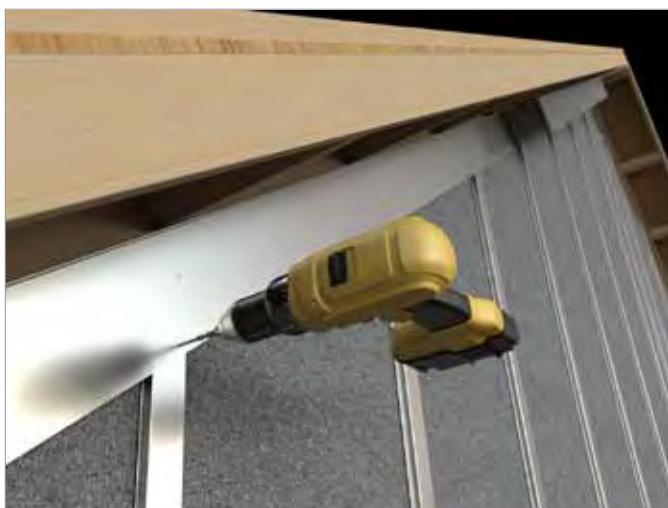
Spandrel - bracing / lateral support
