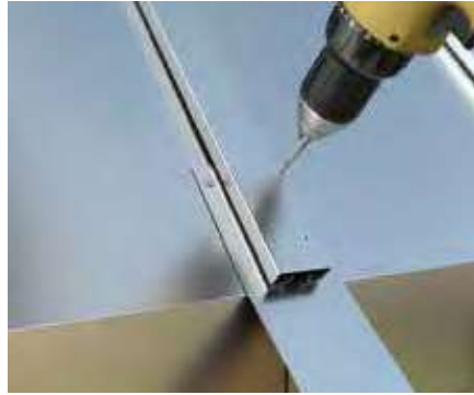
2. Two fixings through the clip and two each side of the soffit where it overlaps onto the roof - 4.2 x 38mm GPHS001
