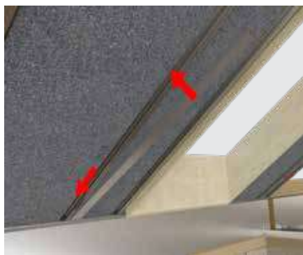
21. Moving inside to fit the steel clips to the underside of the panels. The inner clips are supplied in two pieces – a short length to be used at the eaves and a longer length for the ridge end. At the eaves end, 'spear' the short steel clip onto the roof panel rails, then drive/tap the short clip fully down into the eaves shelf
