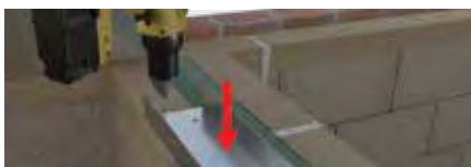
7. Measuring from the cavity side of the wall plate set the back edge of the angle plate inboard by 63mm. Screw down at 300mm centres using 4.2mm x 38mm screws (or 3.1 x 45 ARS nail)
